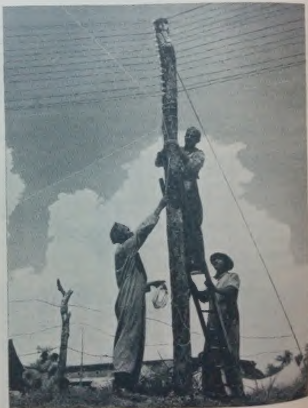
Signalmen laying telephone lines near Naushera.
